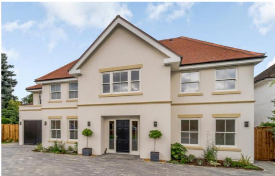
Completed replacement two-storey dwelling opposite the proposed development
