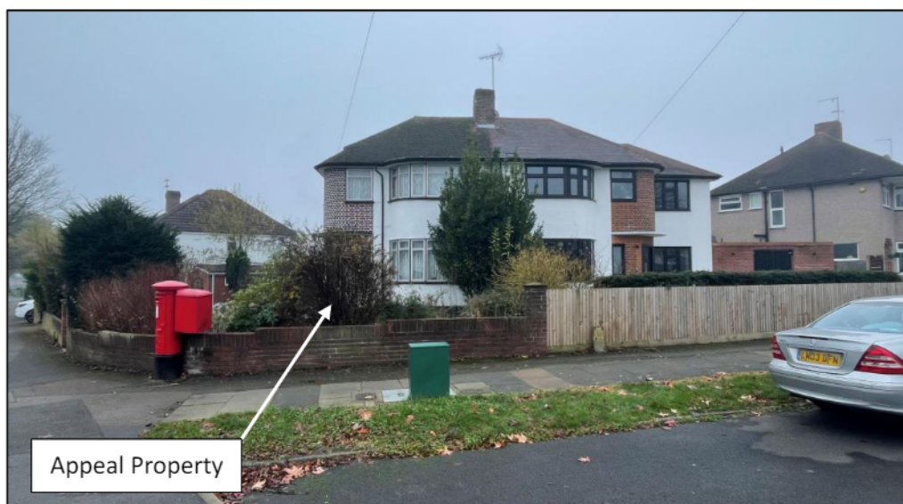
No. 398 Field End Road and No. 1 Ferncroft Avenue
