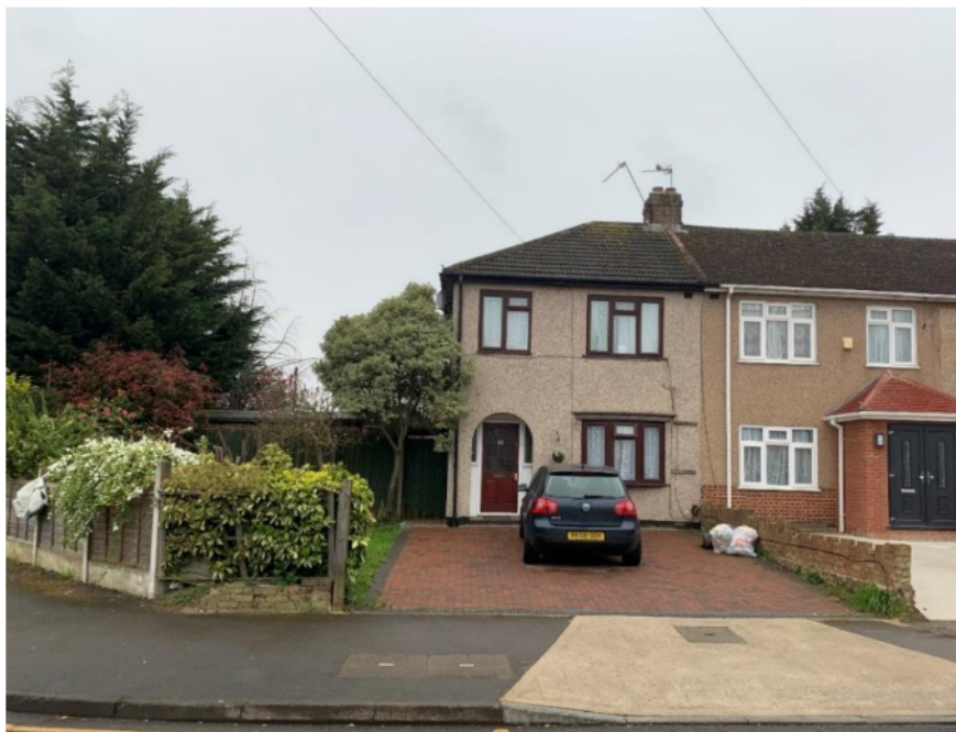
Front View of the Property 82 Willow Tree Lane
