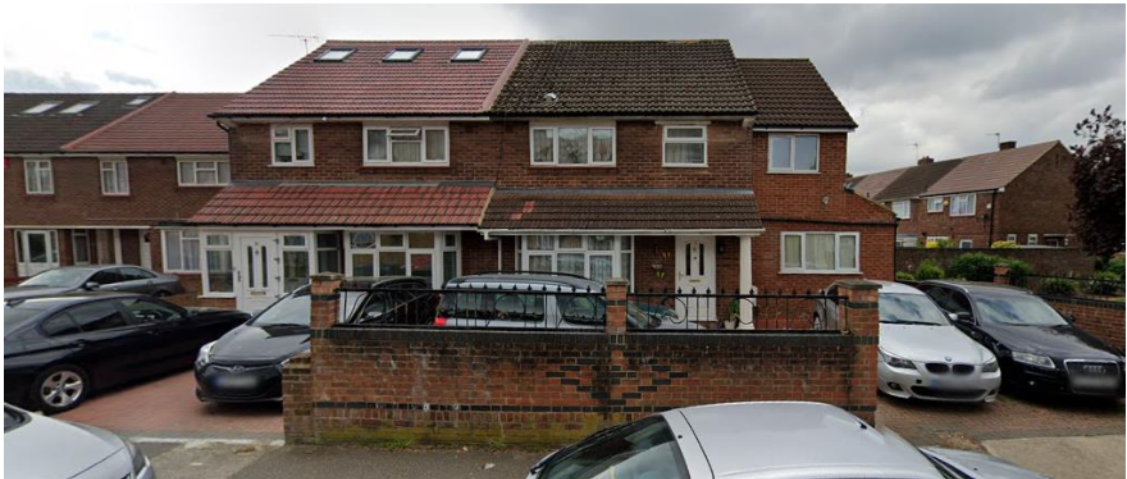
Nos. 11 and 13 Attlee Road prior to appeal development
