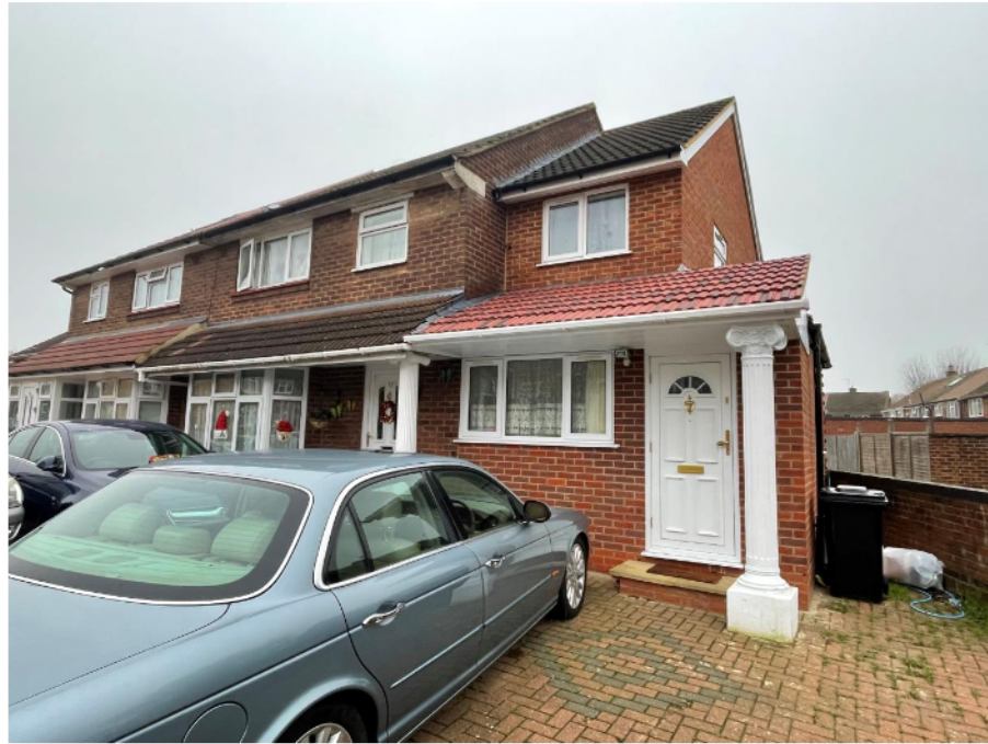
Single storey front extension
