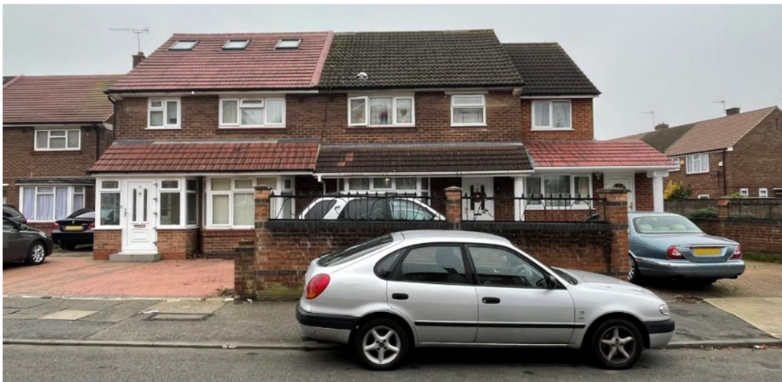
Nos. 11 and 13 Attlee Road post construction of front extension and canopy
