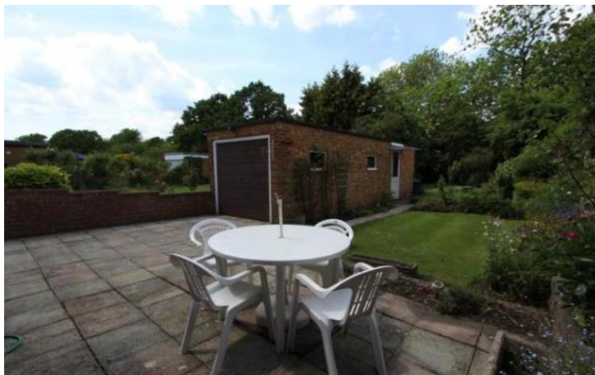
Existing garage to be demolished
