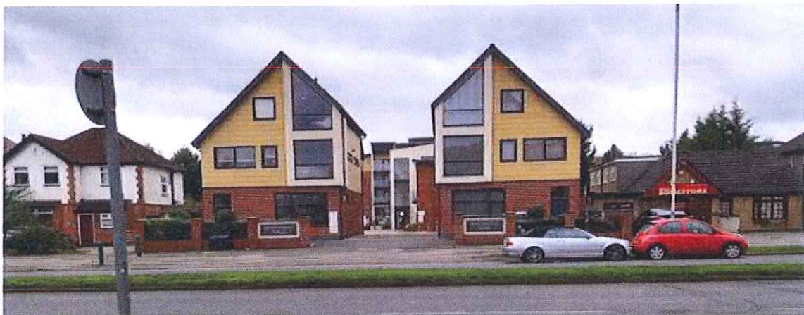
Kingswood Place Uxbridge Road, Hayes as presented in the first photo - Street scene view from the east of the proposed development site 549 Uxbridge Road, Hayes.
