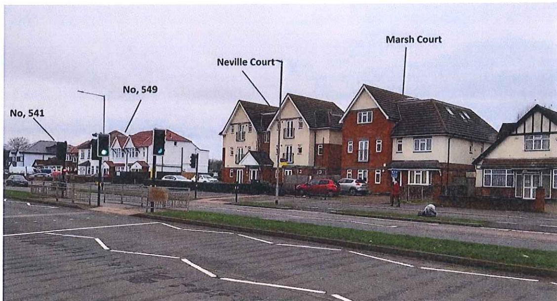
Street scene view from the west of the proposed development site 549 Uxbridge Road, Hayes.
