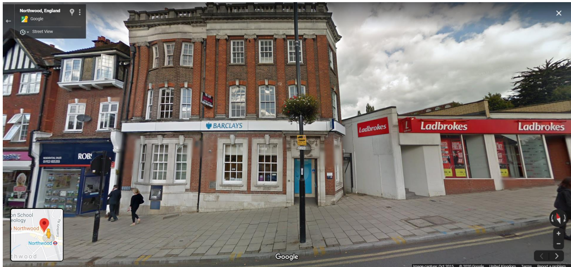
Google Street View Image showing signage on Barclays Bank at opposite end of Green Lane. Building is comparable to appeal site and also locally listed.
