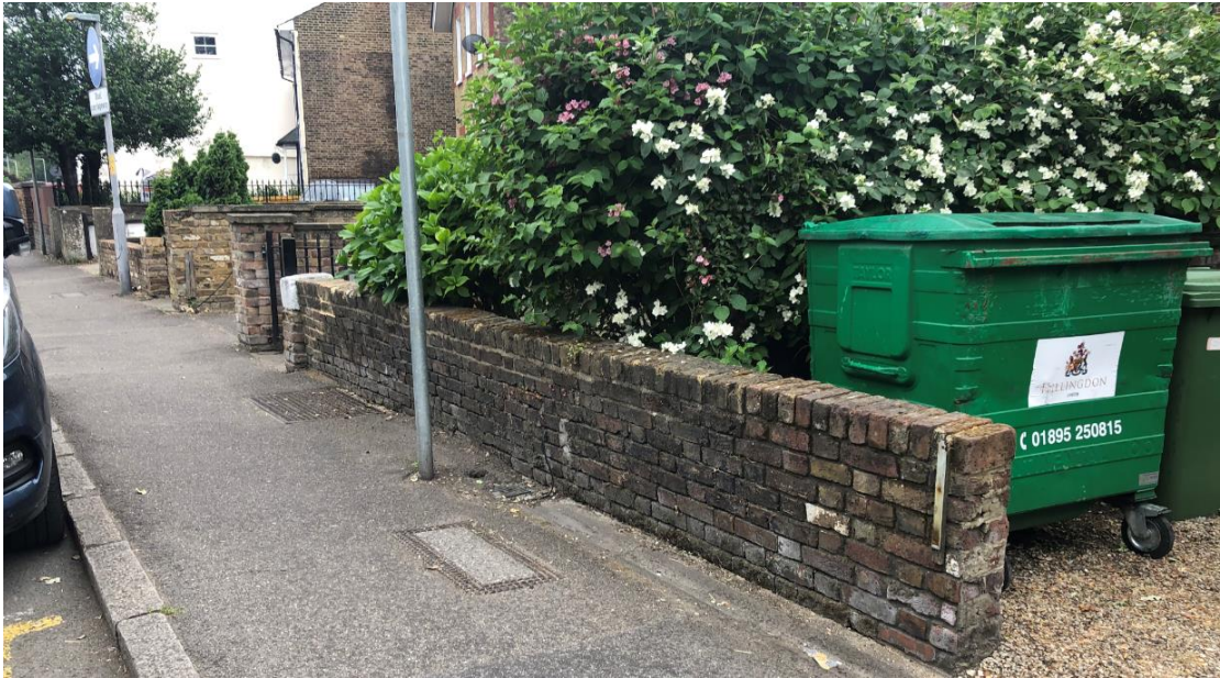
Existing brick wall
