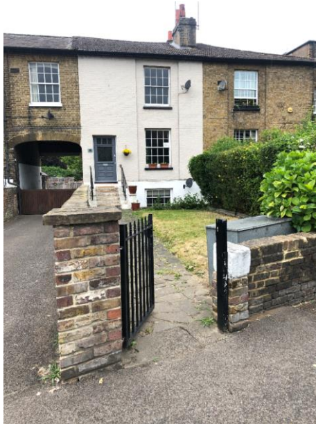
Existing boundary treatments
