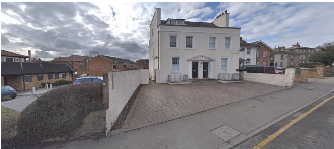
Grade II listed building nos. 11 and 12 Hillingdon Road
