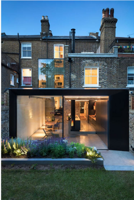
Figure A01: Boscastle Rd, London. Zinc and glass rear extension. The original house was built in a different era for a different type of living. The extension creates a connection to the garden and improves internal flow.
