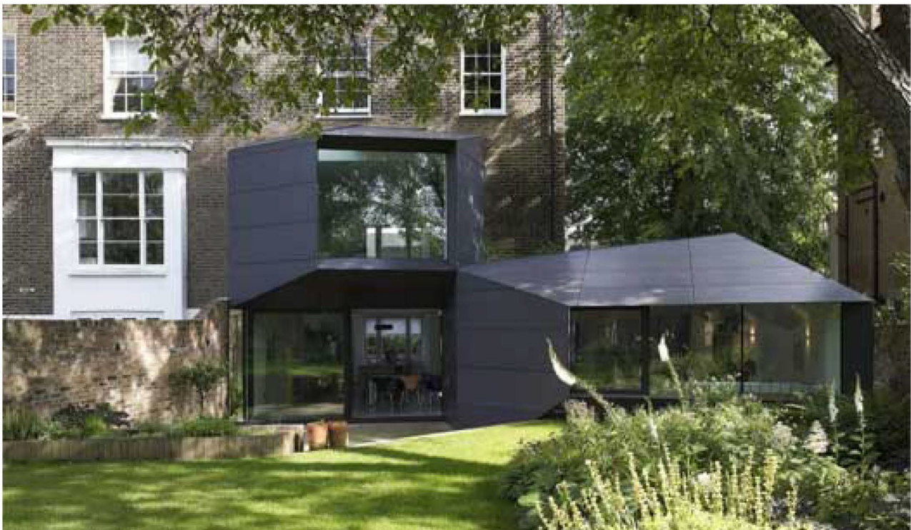
Figure A03: Lens House by Alison Brooks. Contemporary rear extension short-listed for the 2014 Manser Medal. The project involved the conversion of a locally listed 19th Century house in the Canonbury Conservation Area, London.
