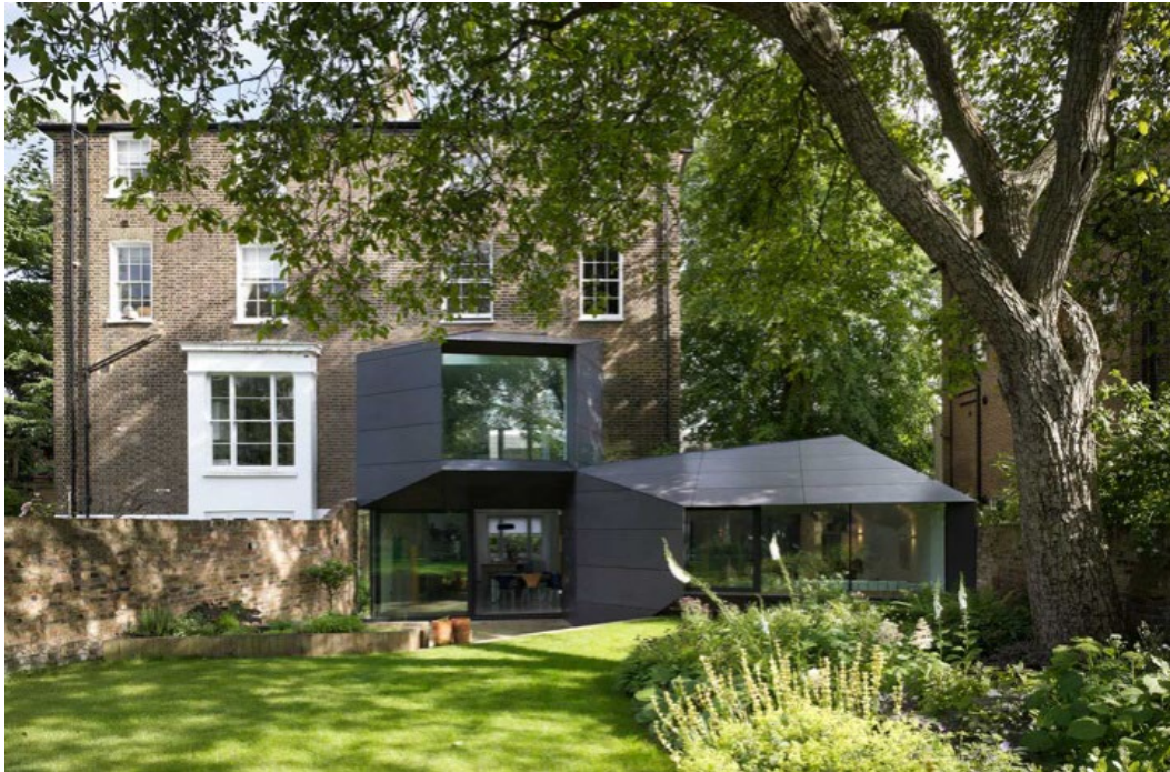
Figure 16: Contemporary zinc extension to a locally listed house in Canonbury Conservation Area
