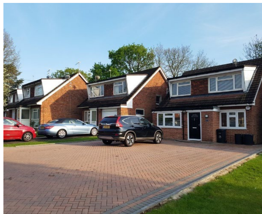
Figure 13: Sylvana Close - Flat-roof dormers
