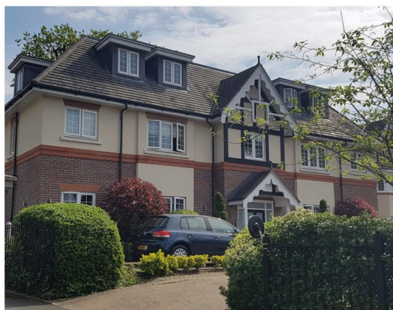
Figure 12: 136 Vine Lane - Flat-roof dormers
