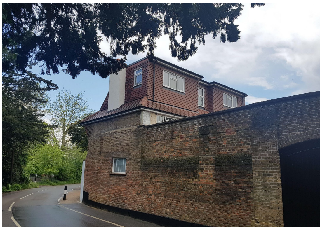
Figure 14: 96 Vine Lane - Flat-roof dormers
