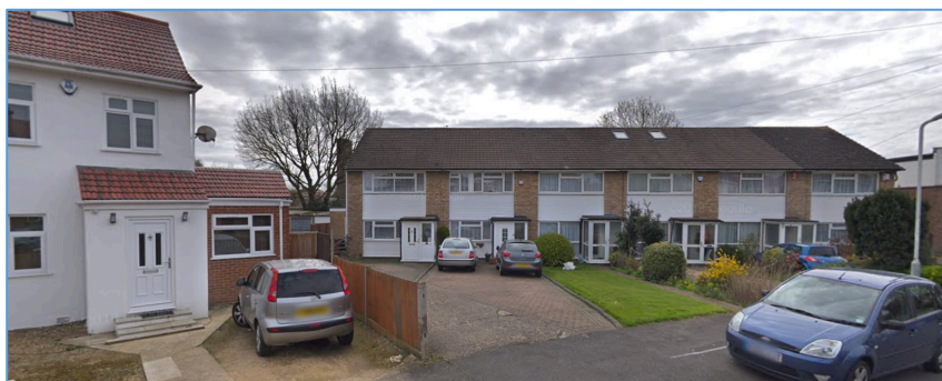
Figure 6: Photograph of front porches at on Dale Drive
