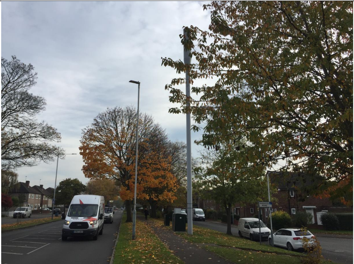
View of the existing mast to the North of Field End Road.
