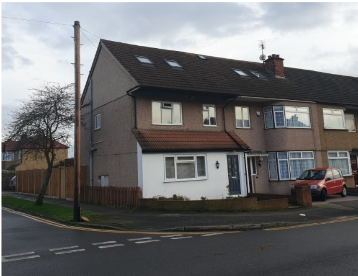
Thurleston Road: No 23A - Roof Style Identical to Proposal of Application
