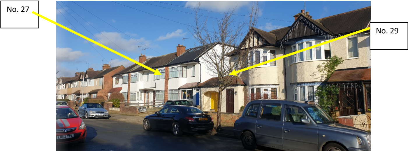
Flamborough Road: Approach From Sidmouth Drive 2
