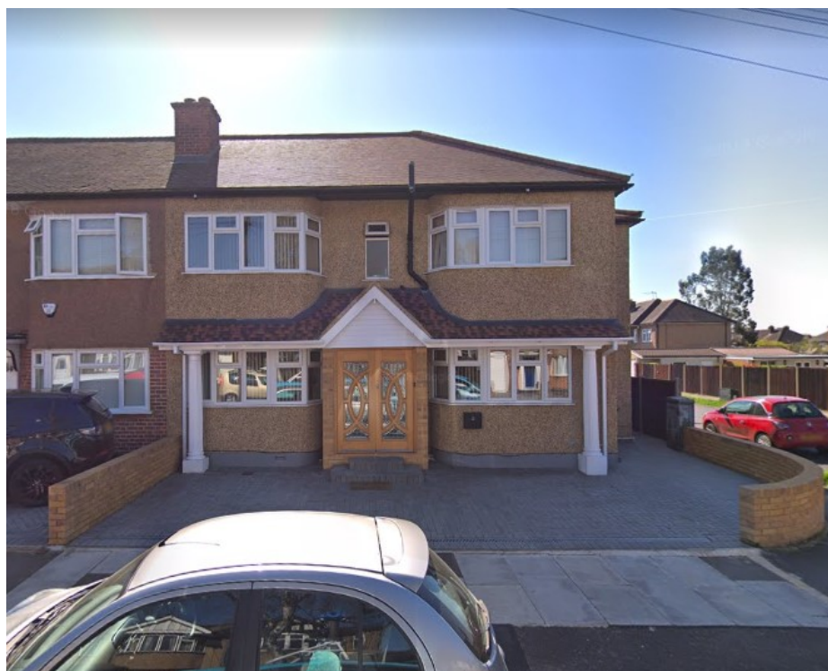
No. 14 Sidmouth Drive: Additional Example of Double Front / Double Bay
