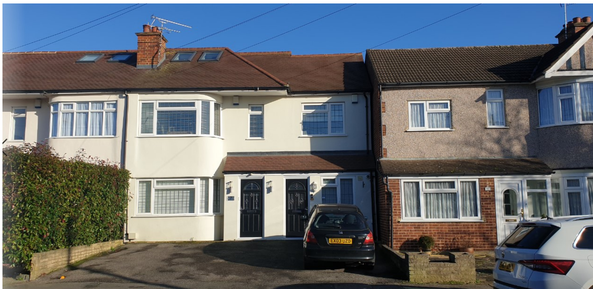
Flamborough Road - No. 7 and 7a , No. 9
