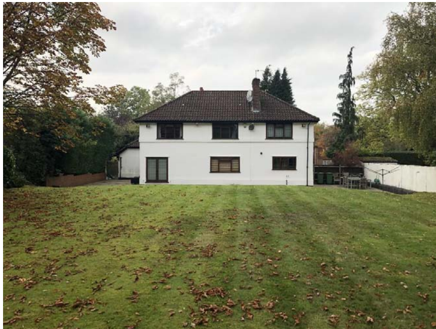
Photograph 2: Existing rear elevation of Five Rivers
