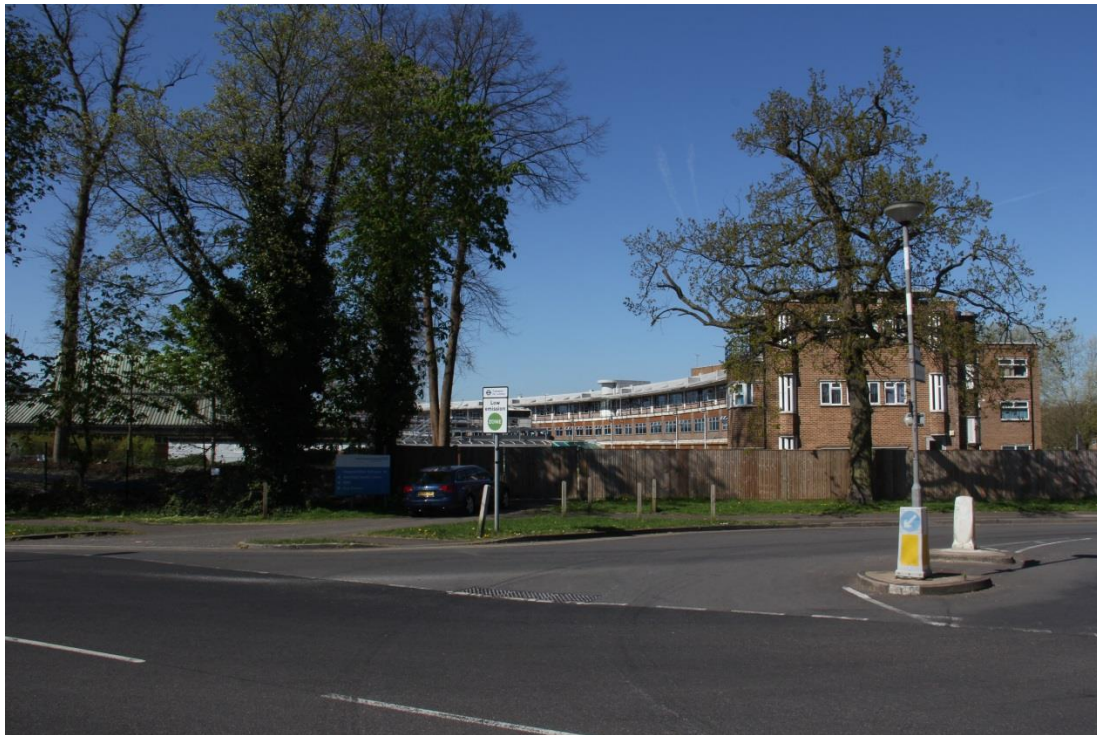
1. 2015 view of site and locally listed hospital building from junction of Rickmansworth Road and Hill End Road.
