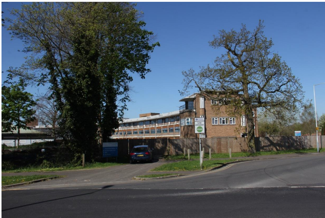
2. 2015 view of site and locally listed hospital building from junction of Rickmansworth Road and Hill End Road.
