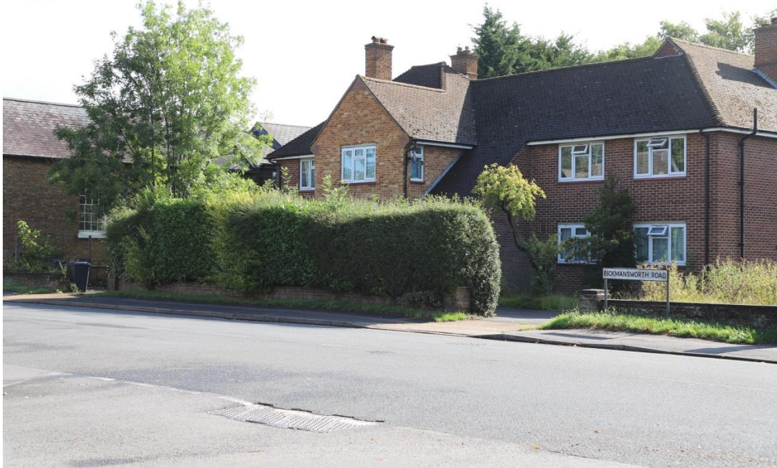
11. 2019 view of no. 24 Rickmansworth Road and the high hedging in front of it.
