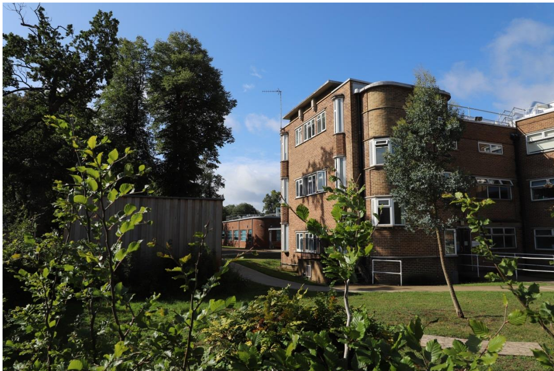
6. 2019 view of locally listed hospital building on right hand side with new store on the left hand side – this shows the setting back of the store, the small scale of the store and the garden area where patients will sit out.
