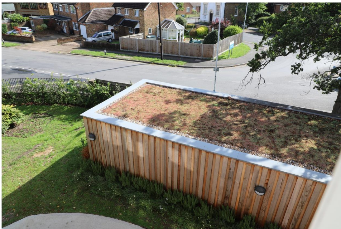
8. 2019 view from the hospital building looking down on the store and its green roof. New low level planting can be seen in the front and Hill End House can be seen beyond.
