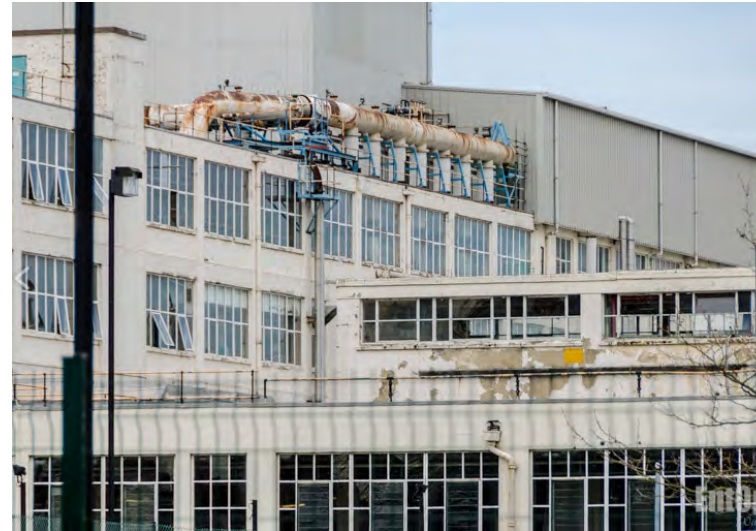
Nestle Factory : Simple industrial blocks with a secondary layer of metal components
