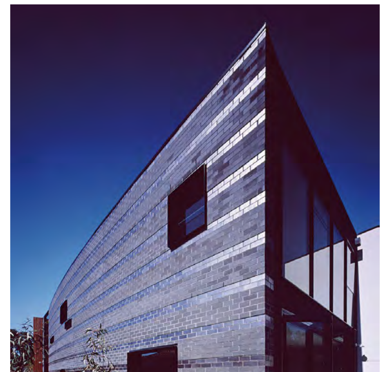
Horizontal facade reading created by smooth and glazed brick bands.
