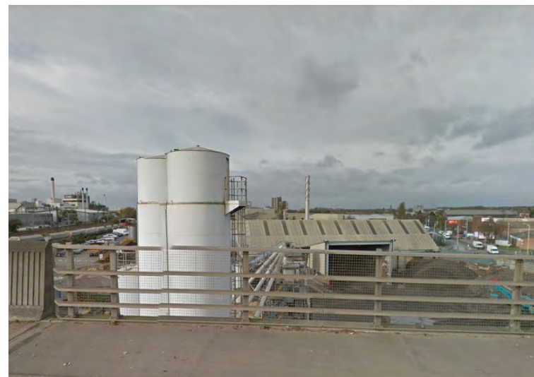
Industrial details of the Tarmac Plant, 2018
