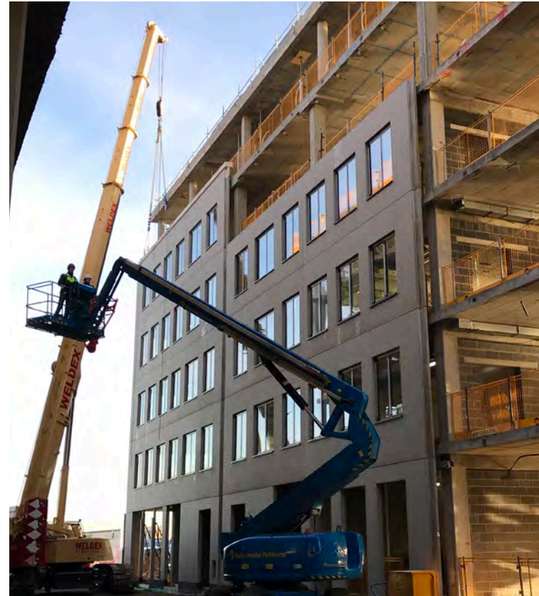
On-site construction of panellised brick façades by Farrells, 2017
