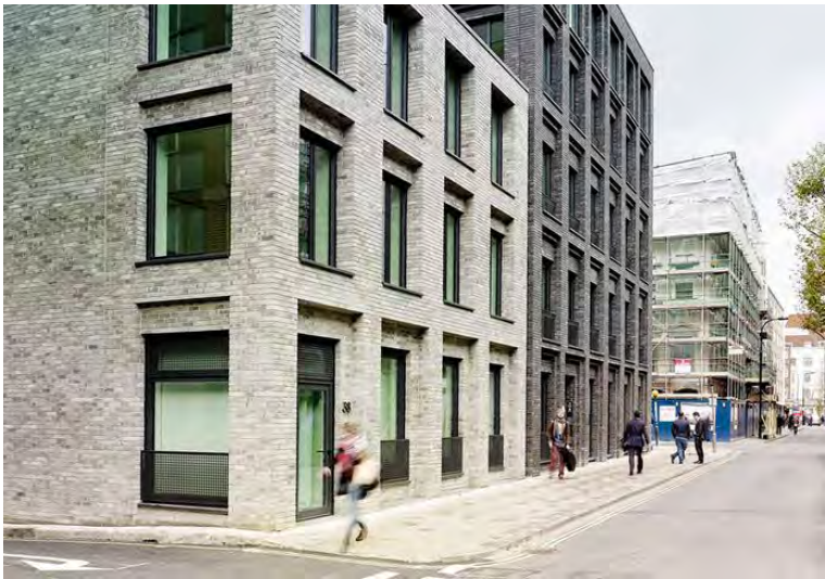
A mixture of brick tones used to define buildings
