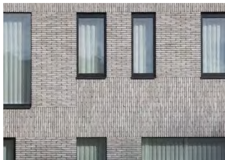
Brick Precedent : Vertical and Horizontal brick courses across a facade
