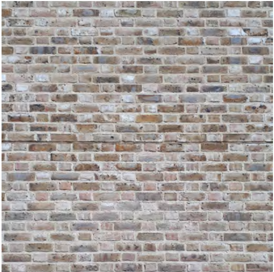
Stock Brick Wall with flush mortar joints
