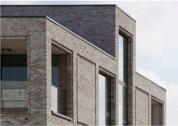
Brick Frames and edges details
