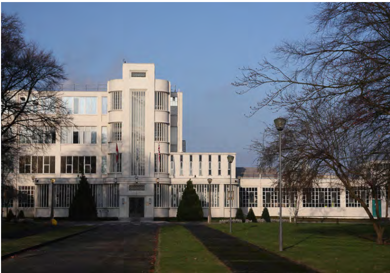
Nestle Factory : Art Deco facade by Wallace, Gilbert and Partners
