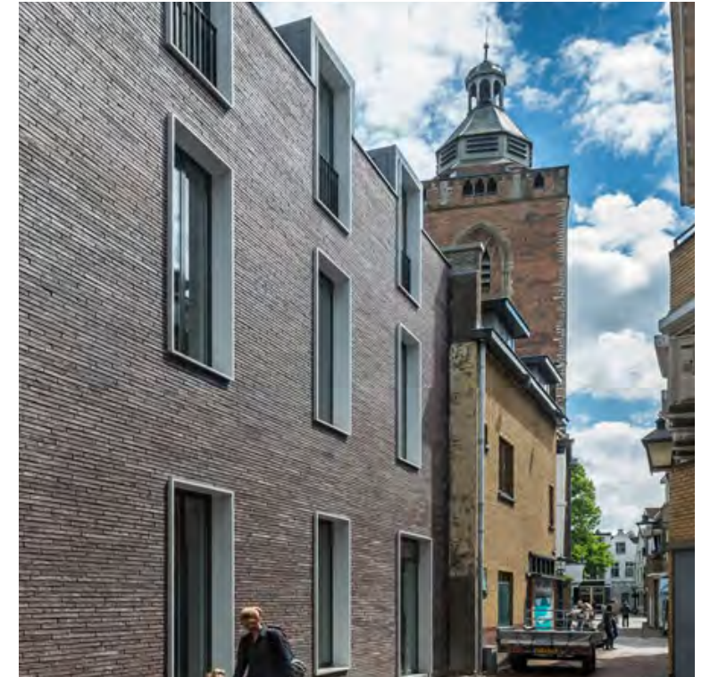
Horizontal brick texture punctured with pronounced window surrounds
