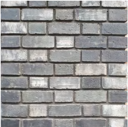
Grey Brick wall with recessed mortar joints
