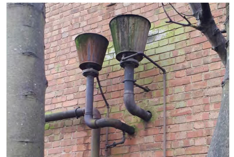
Interesting metal details and brick textures on site, 2017
