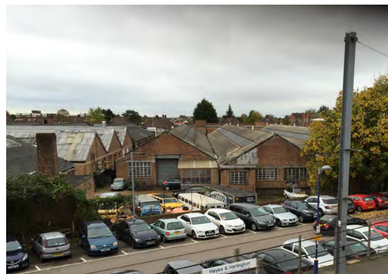
Existing industrial sheds on site, 2017
