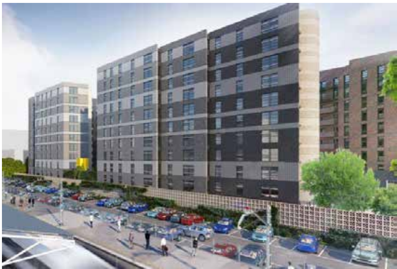
Figure 14 Car Park Boundary Wall (NR)
