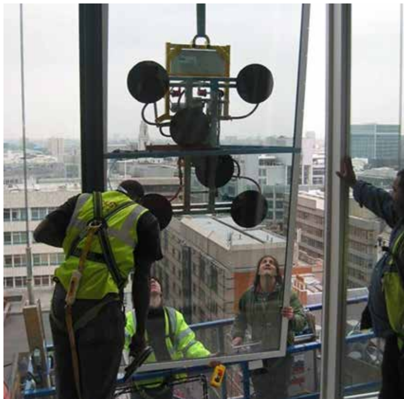
Figure 21 BMU Glass Replacement
