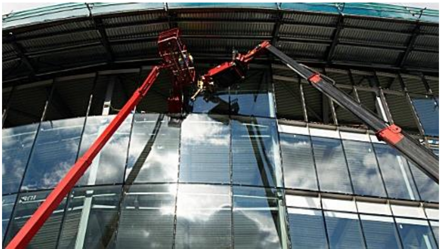
Figure 22 MEWP & UNIC Mini Crane – Glass replacement
