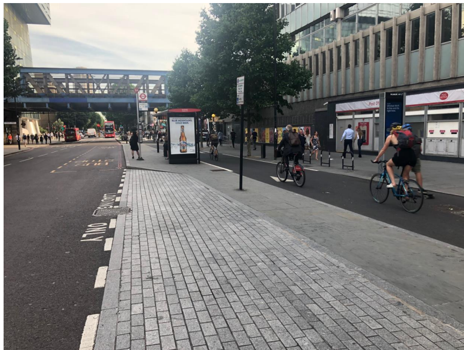
Plate 3.1 – Loading Bay separating Cycle Lane and Carriageway
