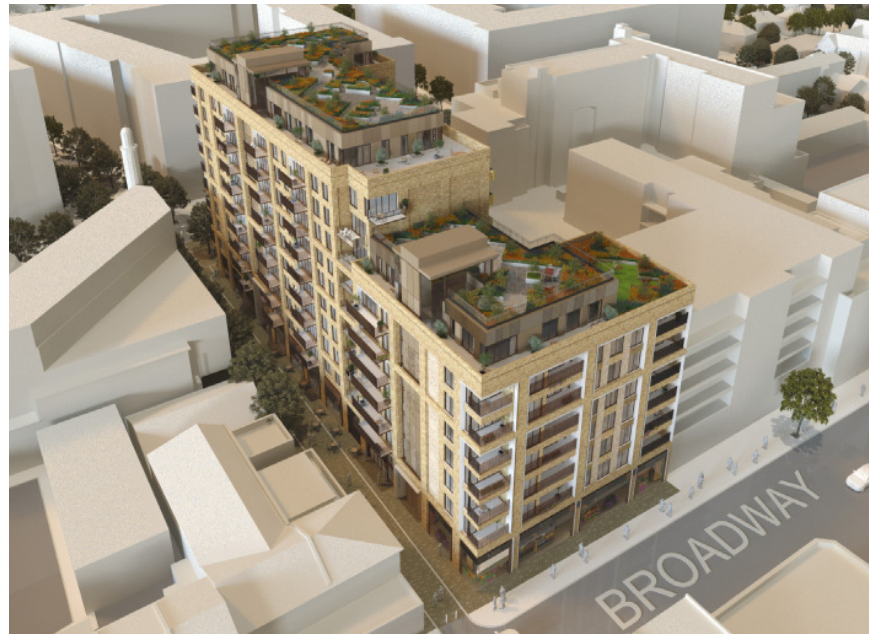
104-110 Broadway, Ealing - Under construction, 136 apartments
