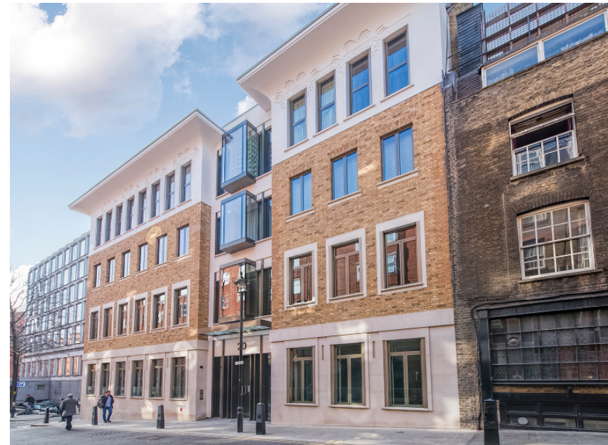
The Hop House, Covent Garden - 30 new apartments
