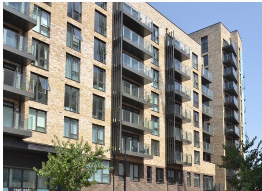
Lansbury Square, Poplar, London - 273 new apartments
