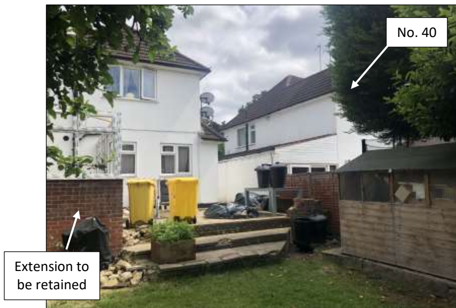
Rear Elevations of Nos. 41-41a and No. 40
