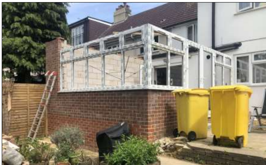
Existing Extension - Partially Constructed at Nos. 41-41a Hillingdon Road
