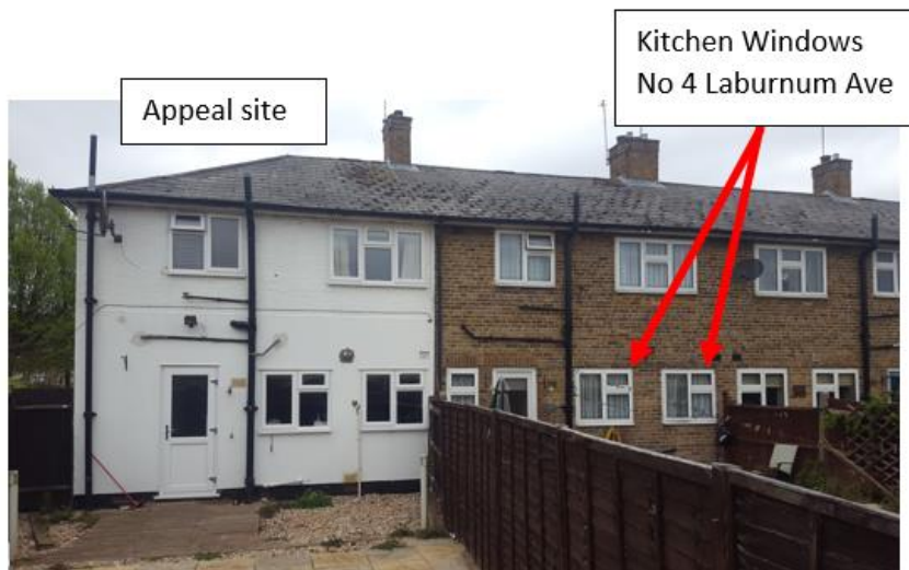
Figure 2 - Photo of rear elevation of Nos 2 - 4 Laburnum Avenue.
