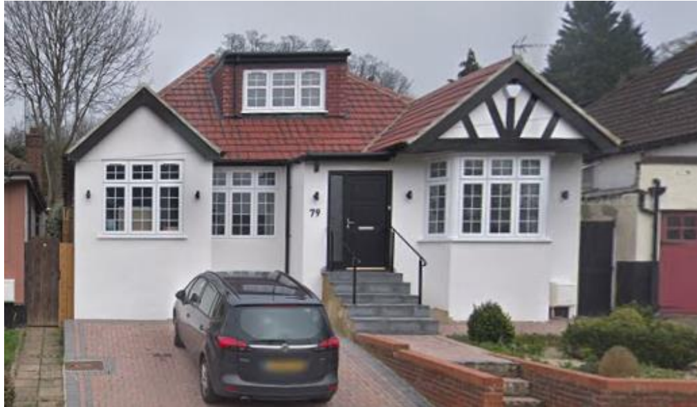
No. 79 Hillside Road prior to and after the completion of approved works
