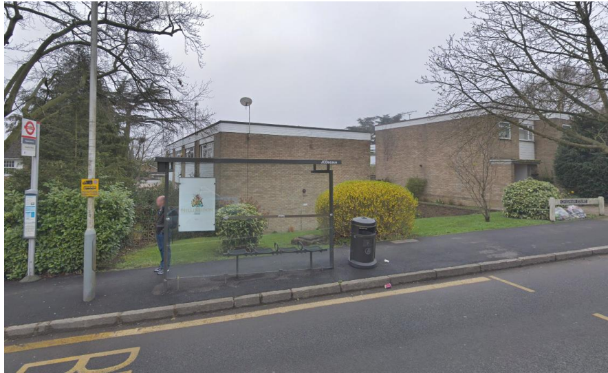
Figure 1 - Chesham Court - directly opposite to the appeal site
