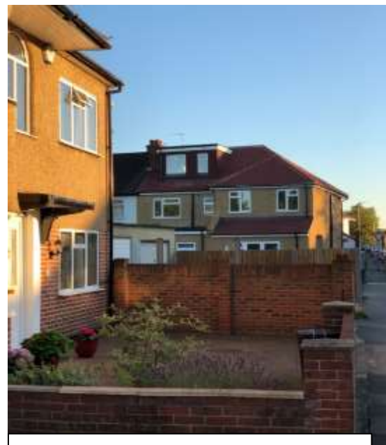
9 Woodlands Avenue, Ruislip- rear
