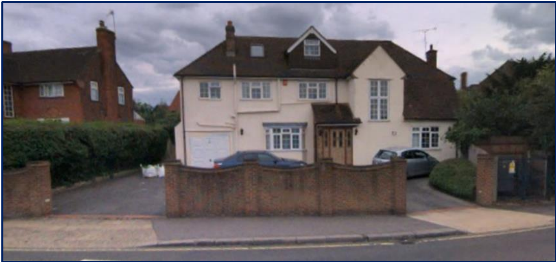
Appeal site No. 51 Ickenham Road
