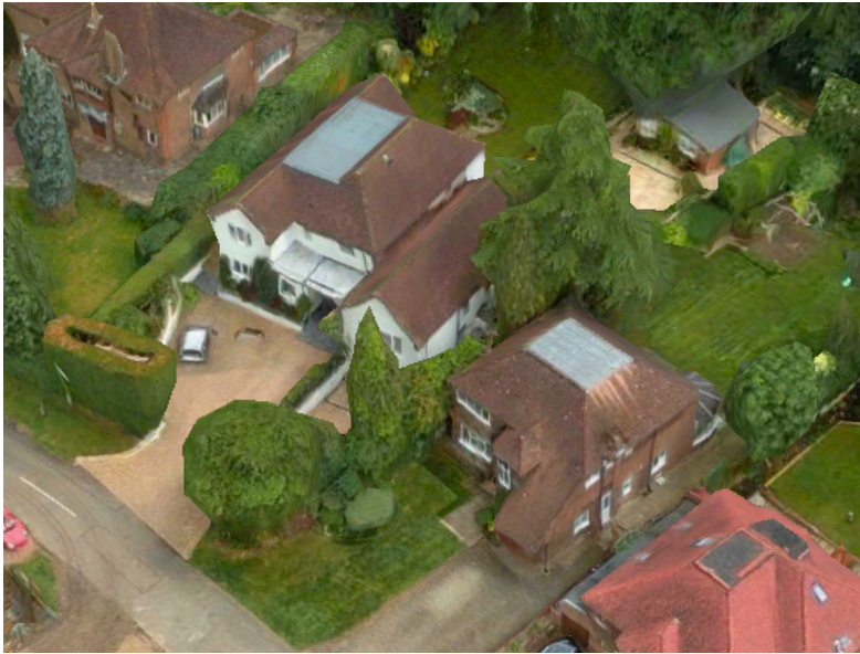
Figure 4 Nos 35 and 37 Wieland Road
