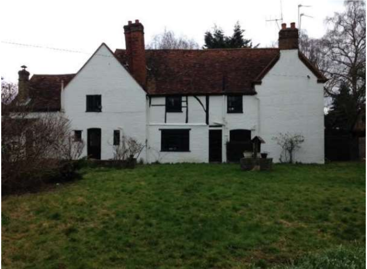
West elevation of neighbouring Listed building
