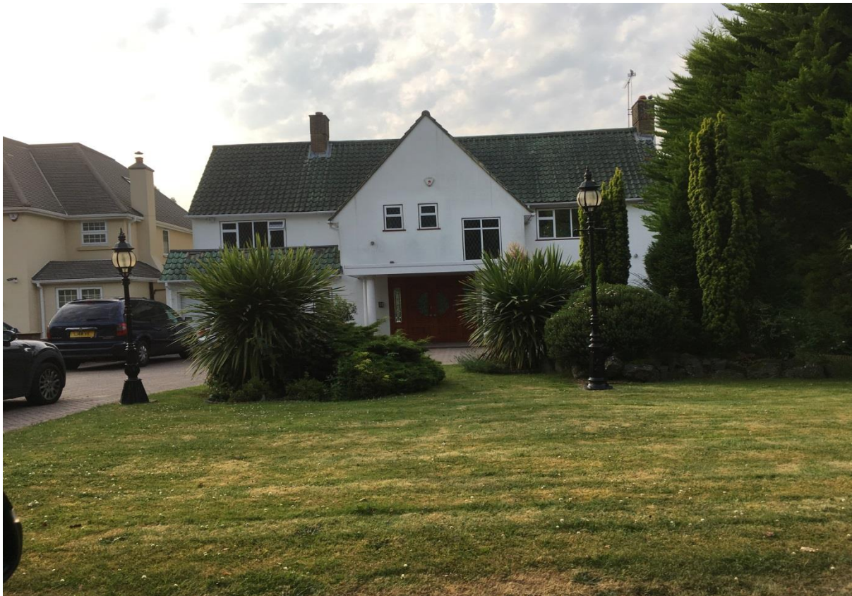
Existing House - 62 The Drive.
