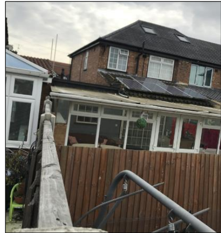
Existing extension at No. 34
