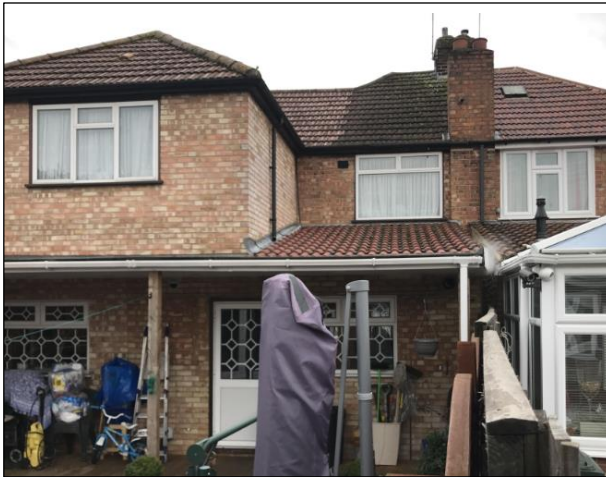
Existing extension at No. 30
