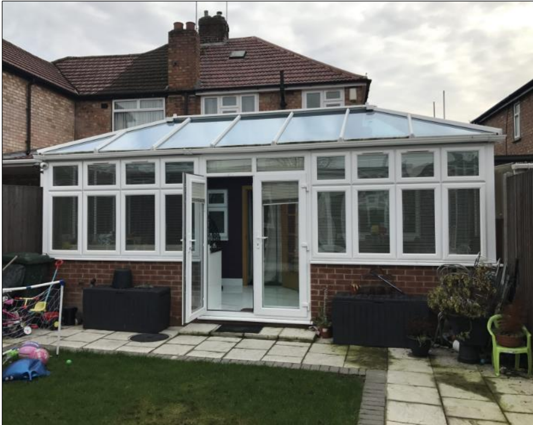
Conservatory to be retained
