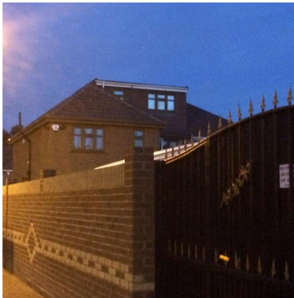
Figure 5 – Rear view of loft extension at 2 Carfax Road, Hayes, UB3. Photo taken on 23/5/16.
