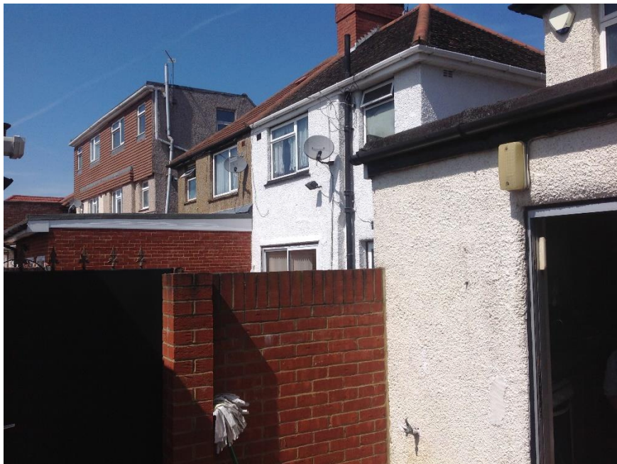
Figure 1 - Rear view of loft extension built at 6 Monmouth Road, Hayes, Middlesex, UB3. The loft extension also adjoins to 8 Monmouth Road. Photo taken on 23/5/16.
