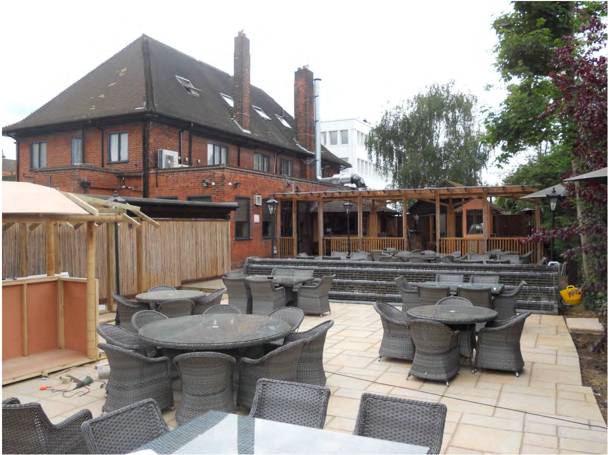
Beer Garden and Rear View of the Main Building
