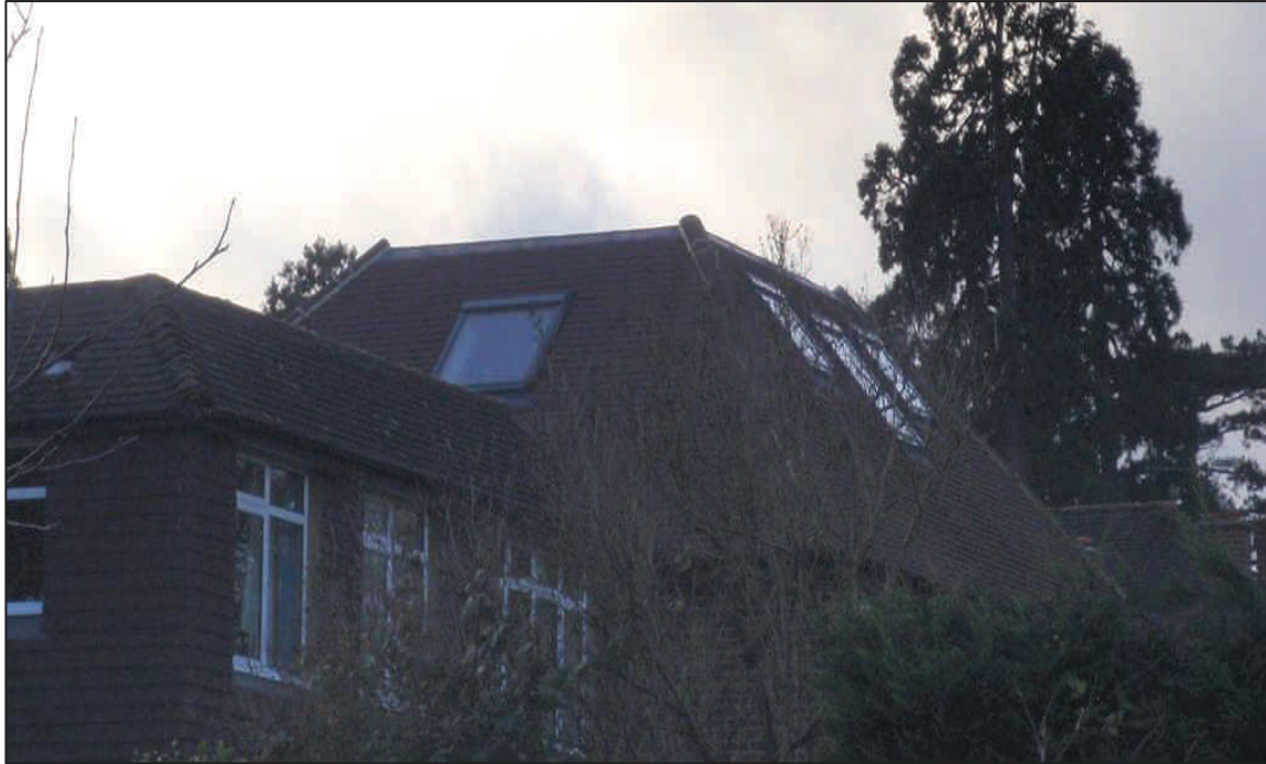
No 47 Warren Road Rear Elevation - Crown Roof Extension
