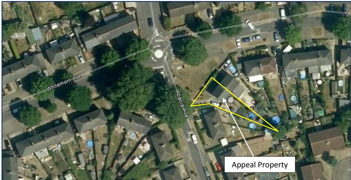
Aerial View of Appeal Site and Surrounding Location
