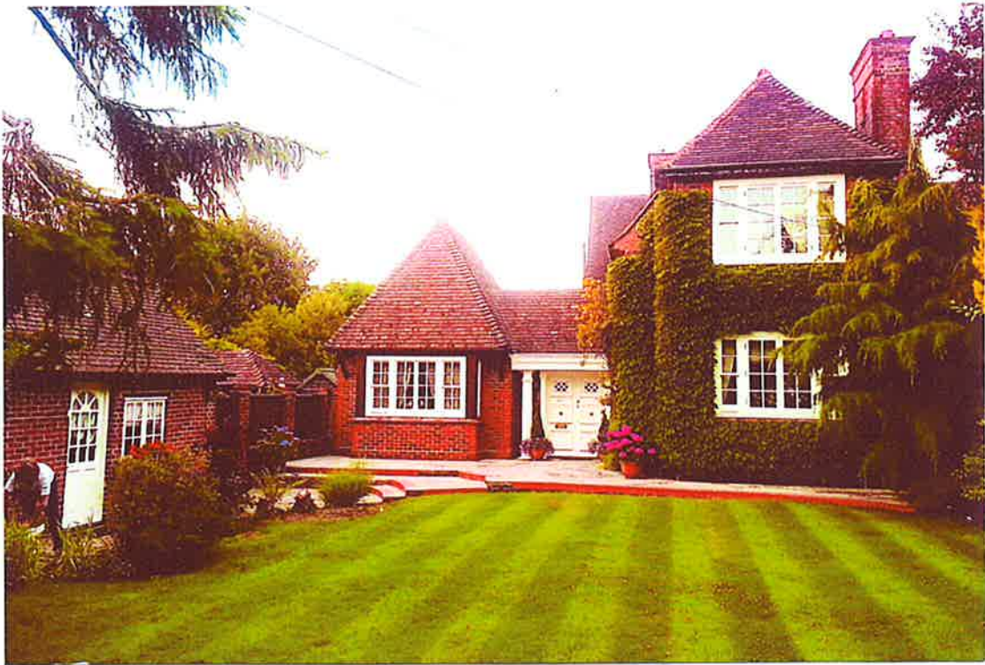
42A WOOD LANE, RUISLIP, MIDDX. SOUTH WEST ELEVATION
