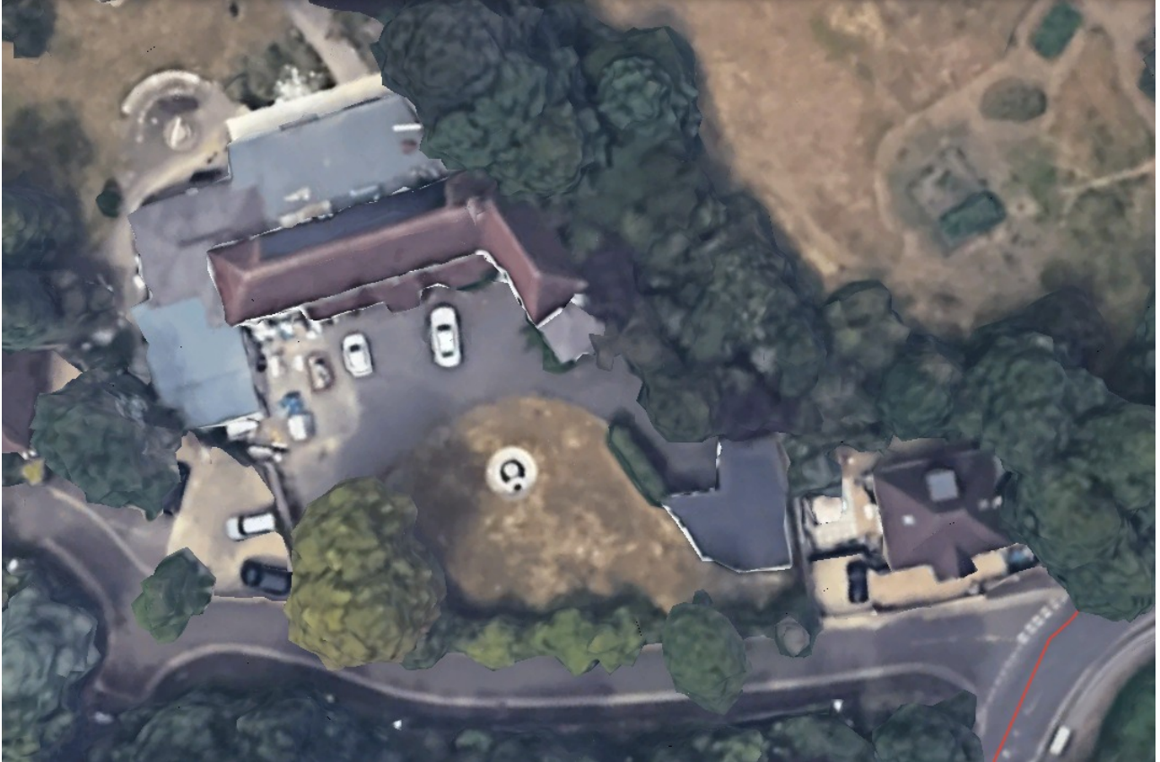
Recent aerial image showing Greensleeves, the outbuilding at the eastern frontage, the common access arrangement and the extensive landscaped site.
