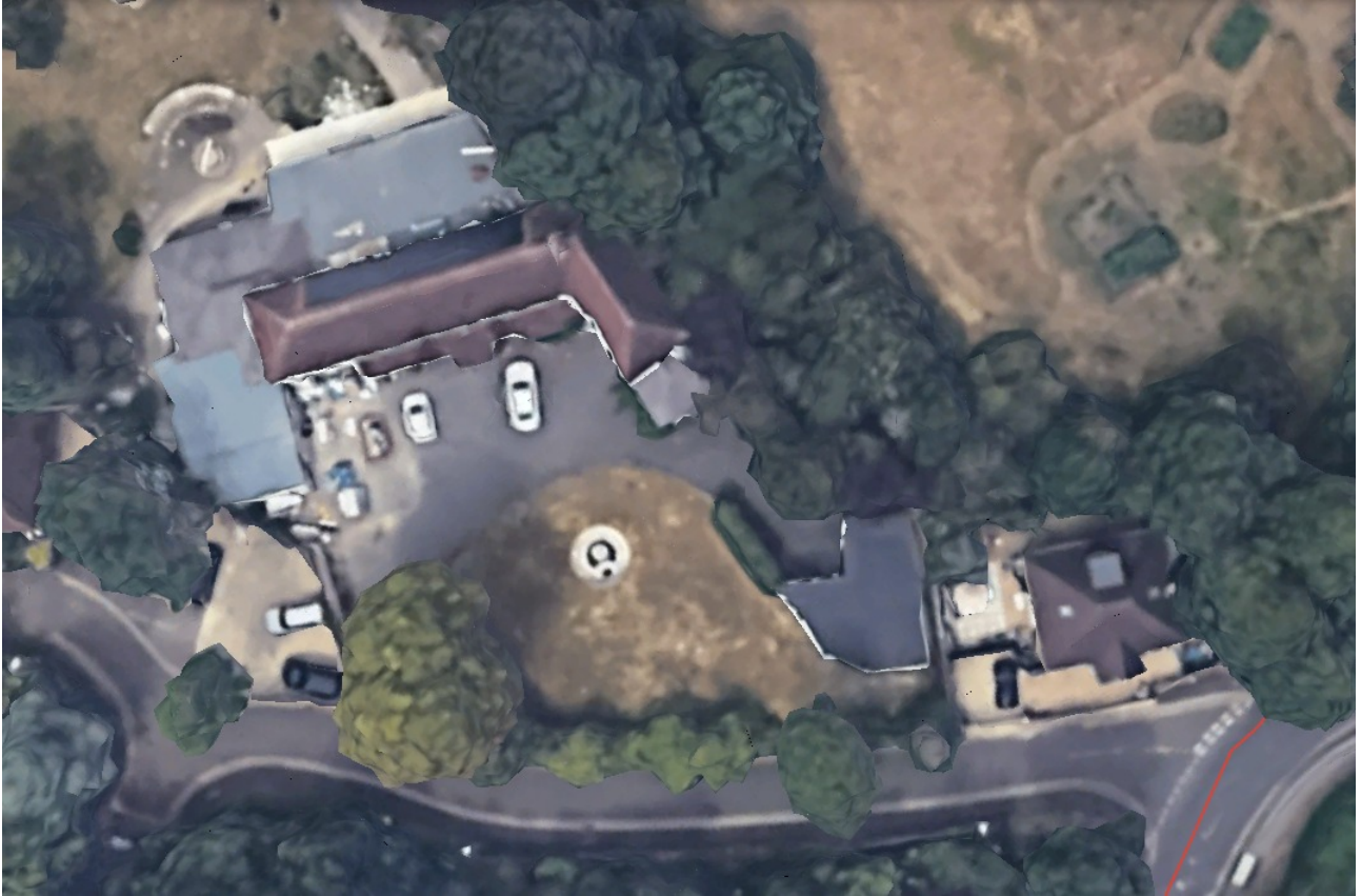
Recent aerial image showing the outbuilding remaining in place and the current wider physical context.
