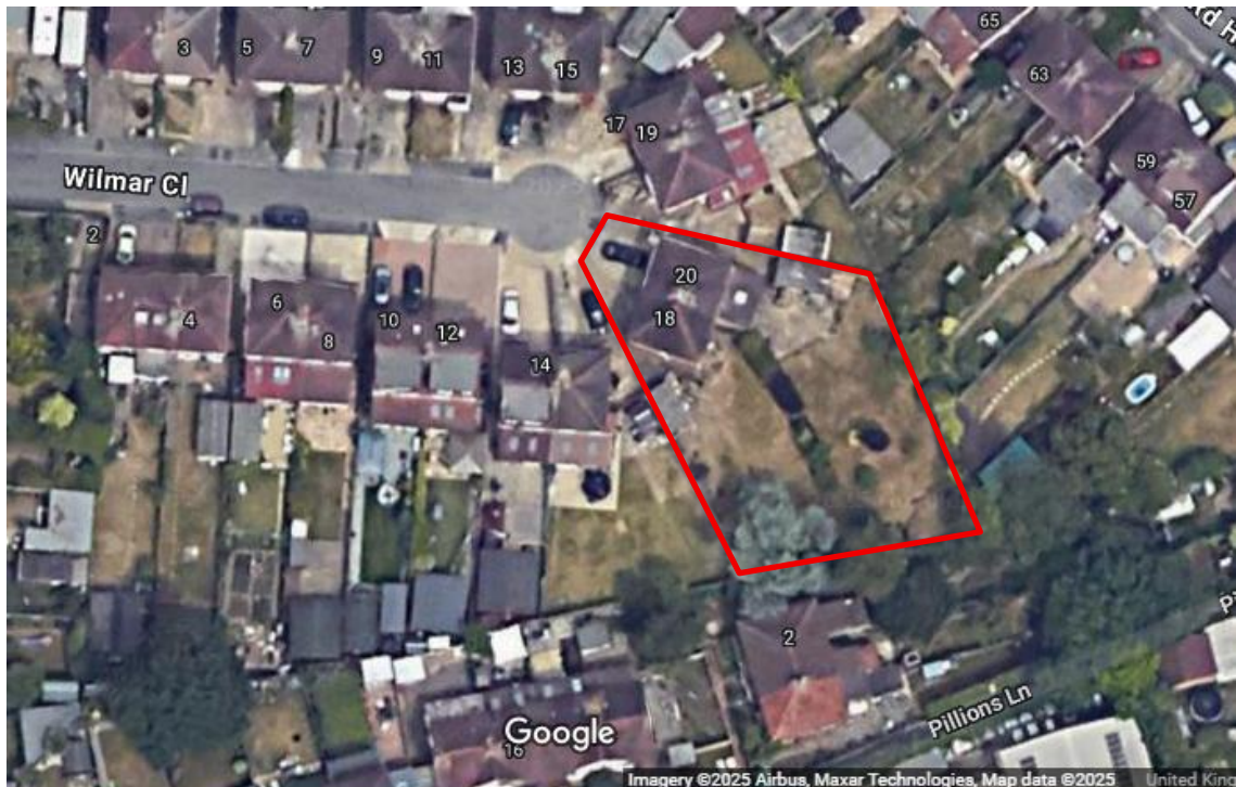
Aerial view of the appeal site
