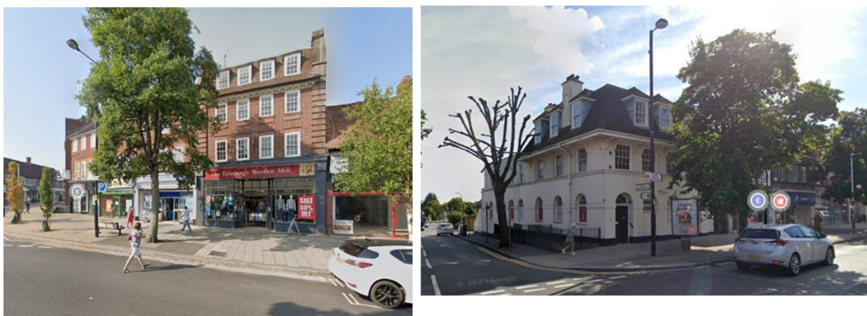
Figure 5: Examples of mansard roofs & traditional dormer windows in the High Street. Source: Google Streetview
