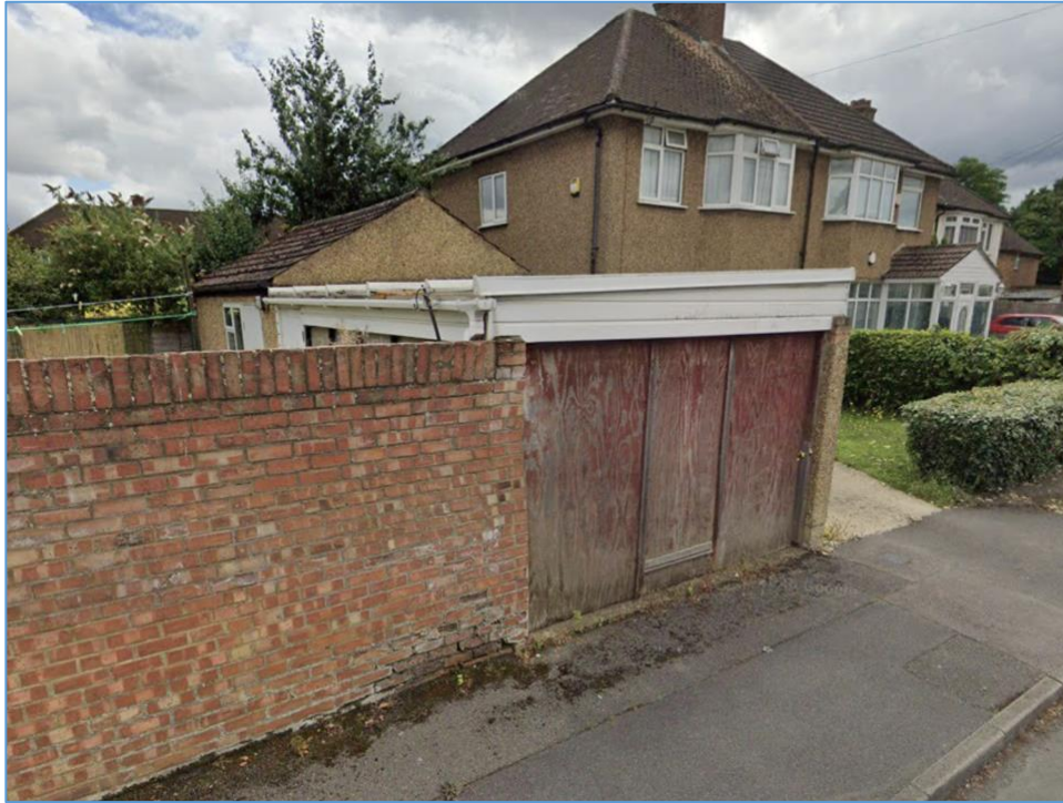
Figure 2: Image of the outbuilding at the rear of the site.
