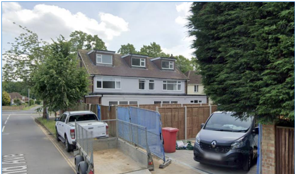
Figure 4: Rear dormers at 30 Long Lane, visible from Almond Avenue.
