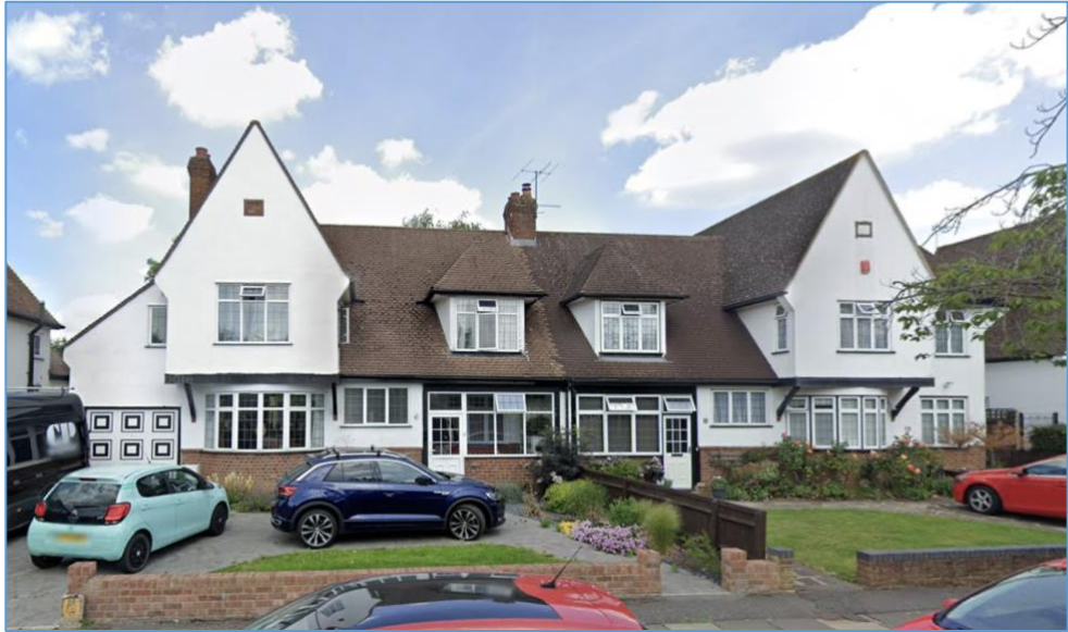
Figure 3: Dormers on houses very close to the appeal site.
