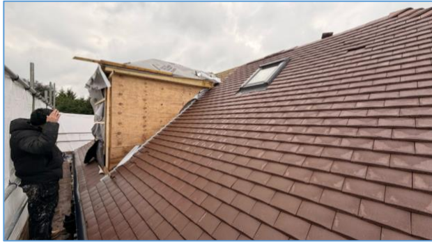
Figure 2: Photograph of one of the dormers.
