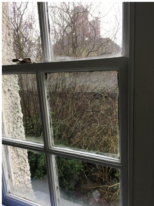
Photograph 5 - First floor side window to Sadie's bedroom
