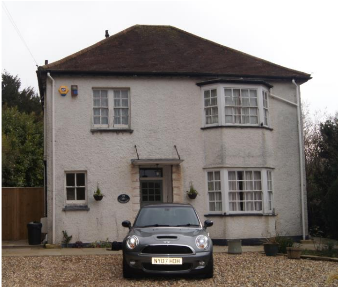
Photograph 4 - Front facade of 17 Elgood Avenue
