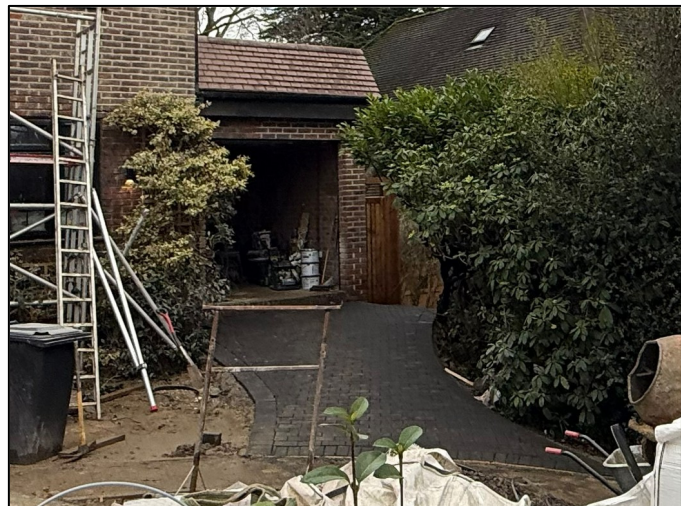
Section of Block Paved Driveway near New Garage
