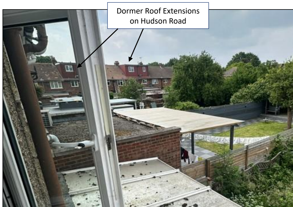
Rear Dormers viewed from the Appeal Property
