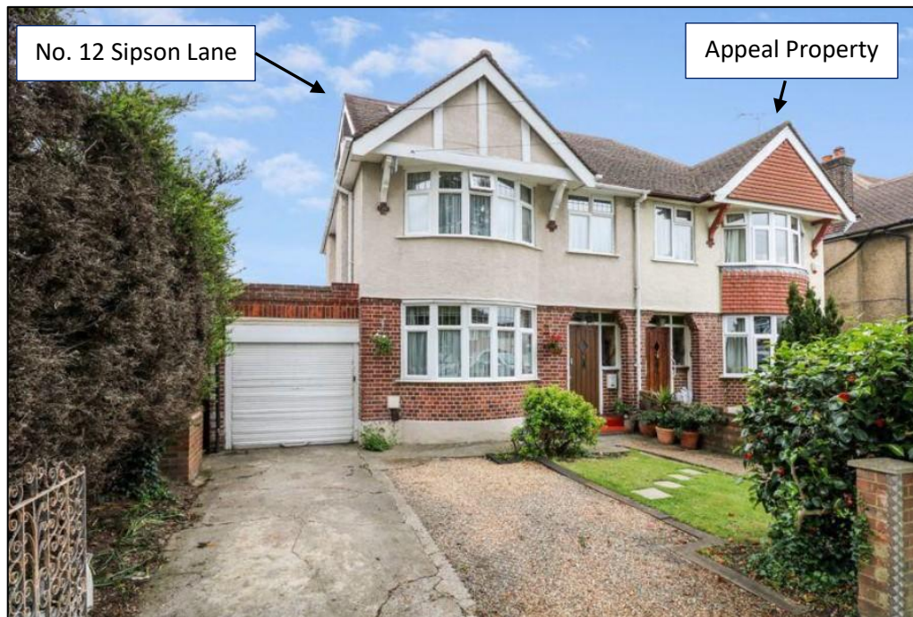
Paired Properties at Nos. 10 & 12 Sipson Lane
