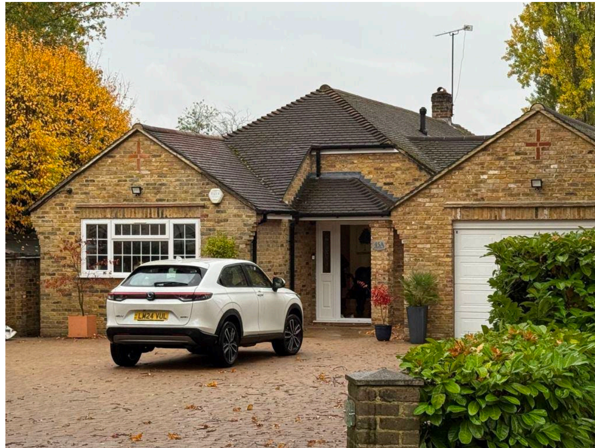
Photographs Showing Neighbouring Properties Along Sweetcroft Lane With Front Projections
