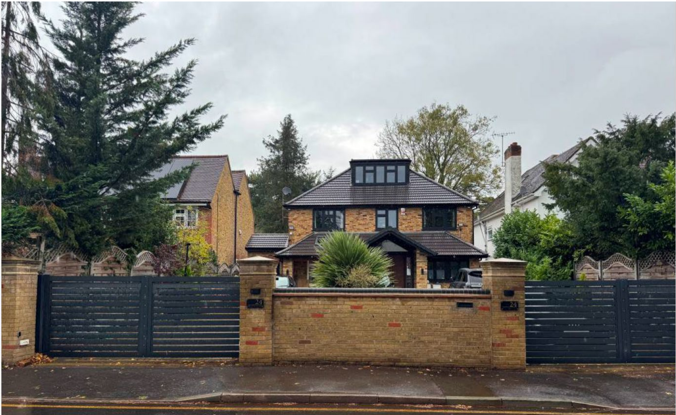
FIGURE 2 Photographs Showing The Existing / As Built Front Elevation Of Number 24 And Neighbouring Properties at Number 22 and 26 Viewed From Sweetcroft Lane
