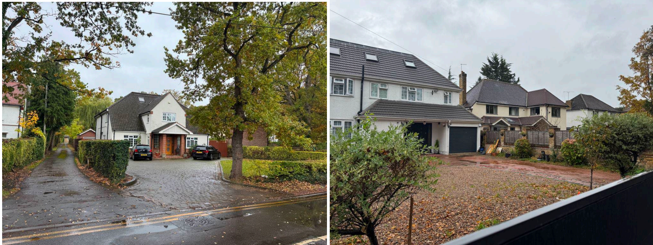
Photographs Showing Neighbouring Properties Along Sweetcroft Lane With Front Projections
