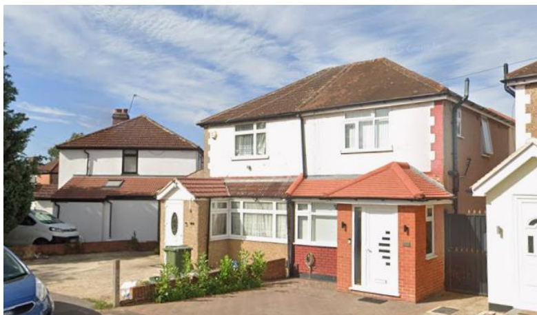
Figure 1 - Front elevation of appeal property
