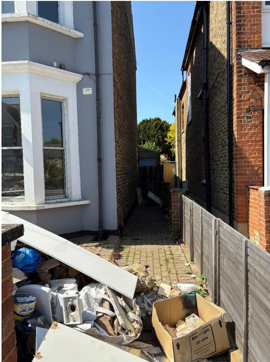
Figure 2: View of Front of 6 Brandville Road
