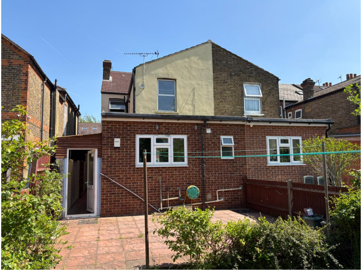
Figure 3: View of Rear Elevation of 6 Brandville Road
