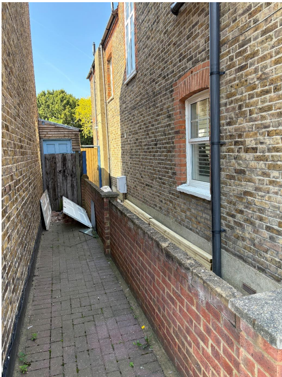
Figure 2: View of Later Side Extension to dwelling and side elevation of 4 Brandville Road
