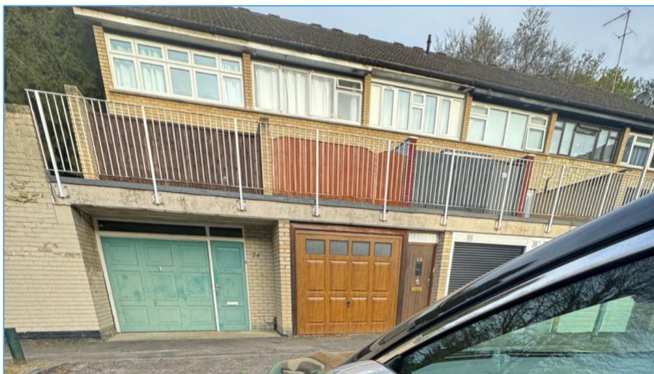
Figure 6: Alterations at Sanctuary Close.
