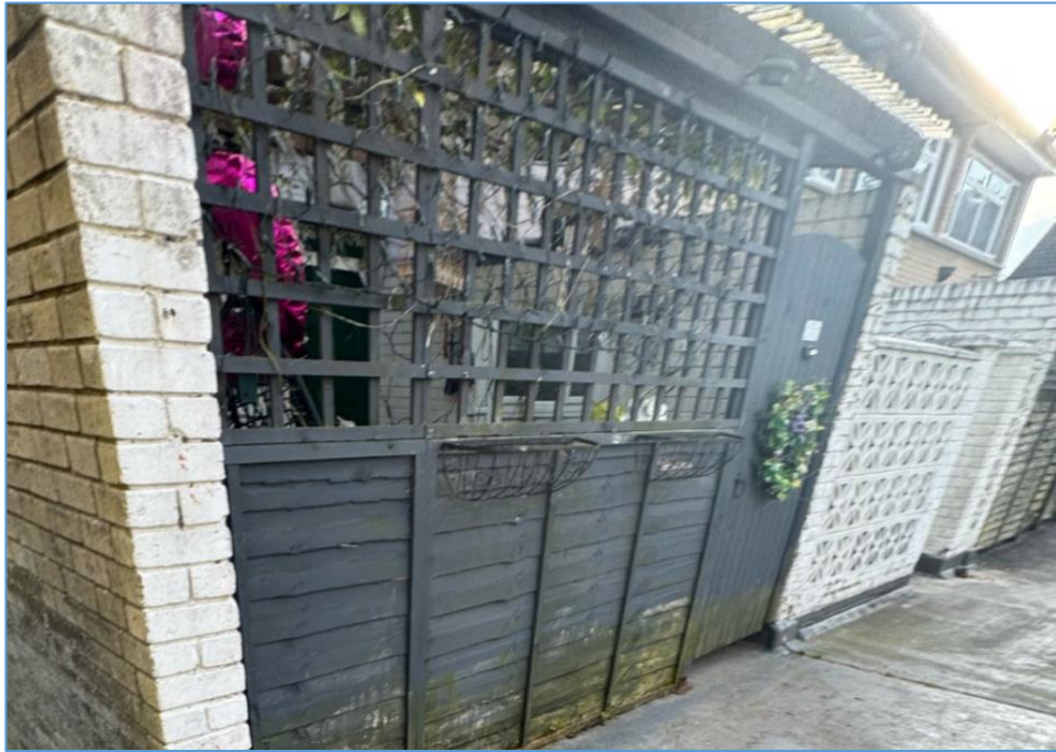
Figure 7: Alterations at Sanctuary Close.
