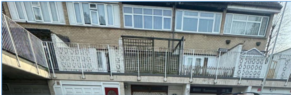
Figure 5: Alterations at Sanctuary Close.
