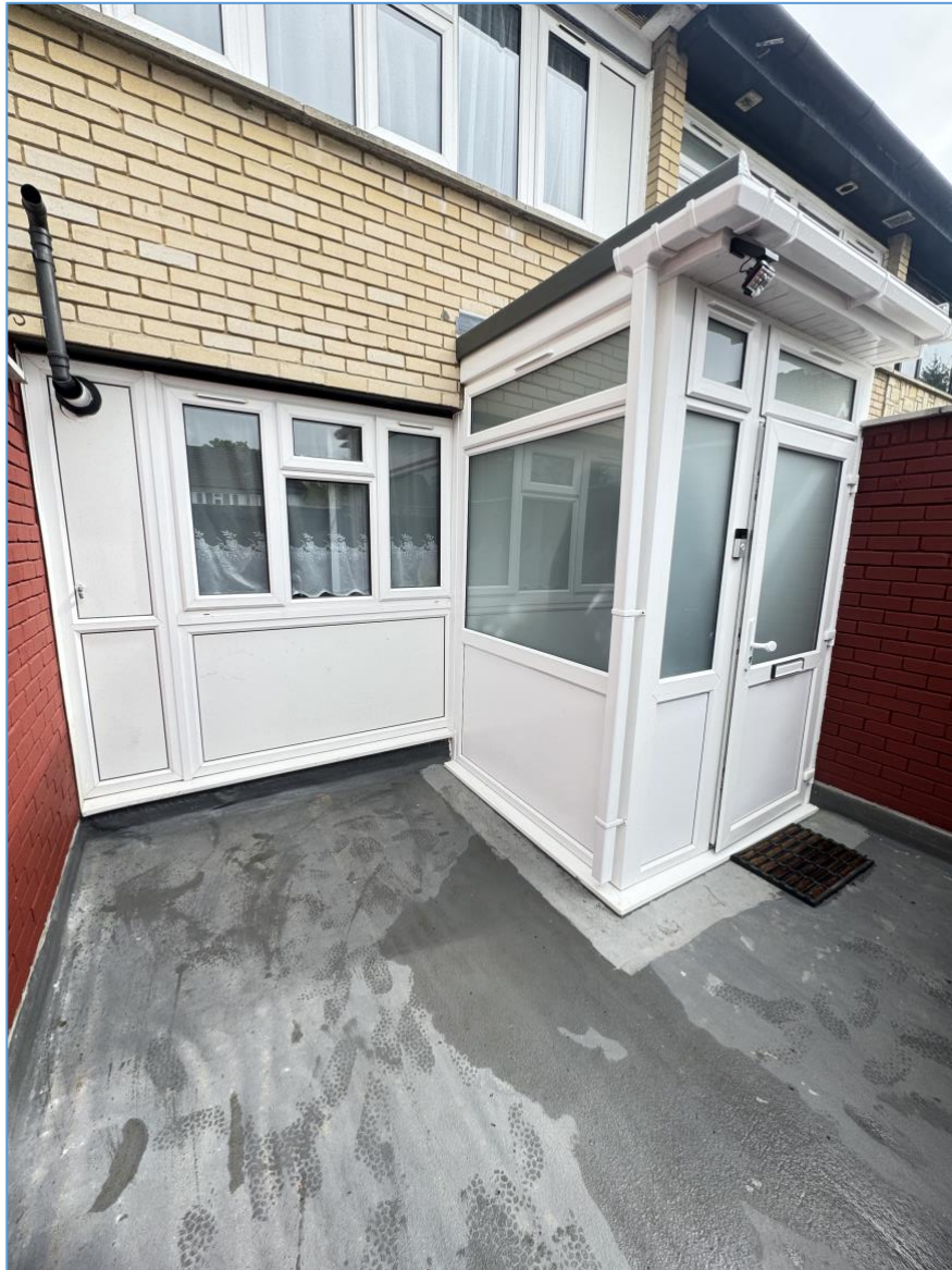
Figure 3: Image of the porch that has been built.
