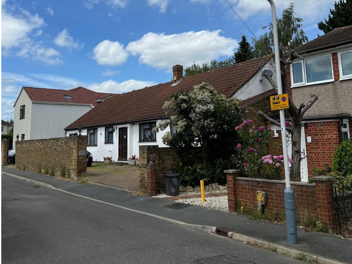
The existing property at 1 Alpha Road in context
