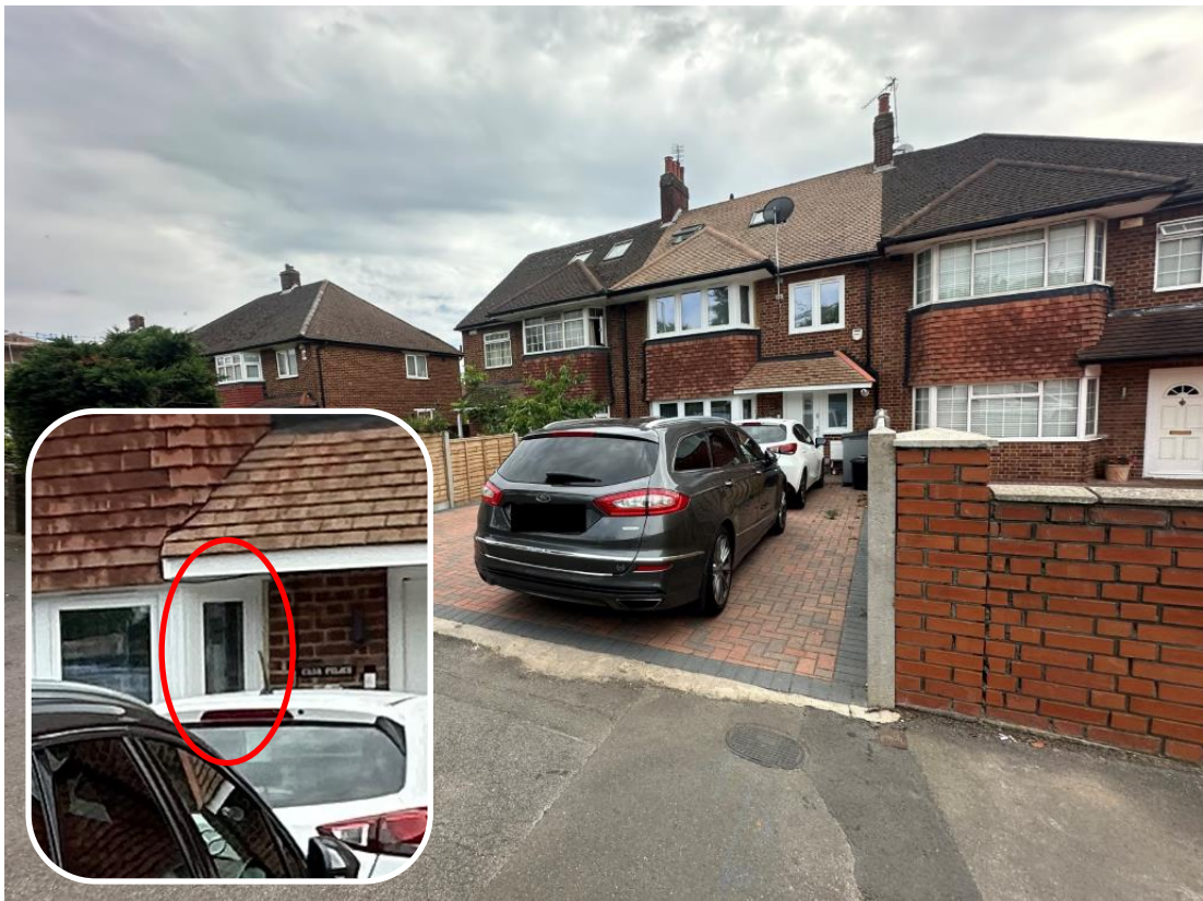
Side facing window (inset) could be obscure glazed or privacy panel installed
