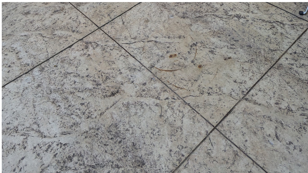
Imprinted concrete finish used as an overlay on top of the pre-existing concrete floor
