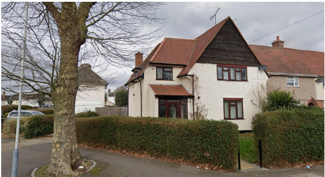
Existing extension at no. 65 Central Avenue
