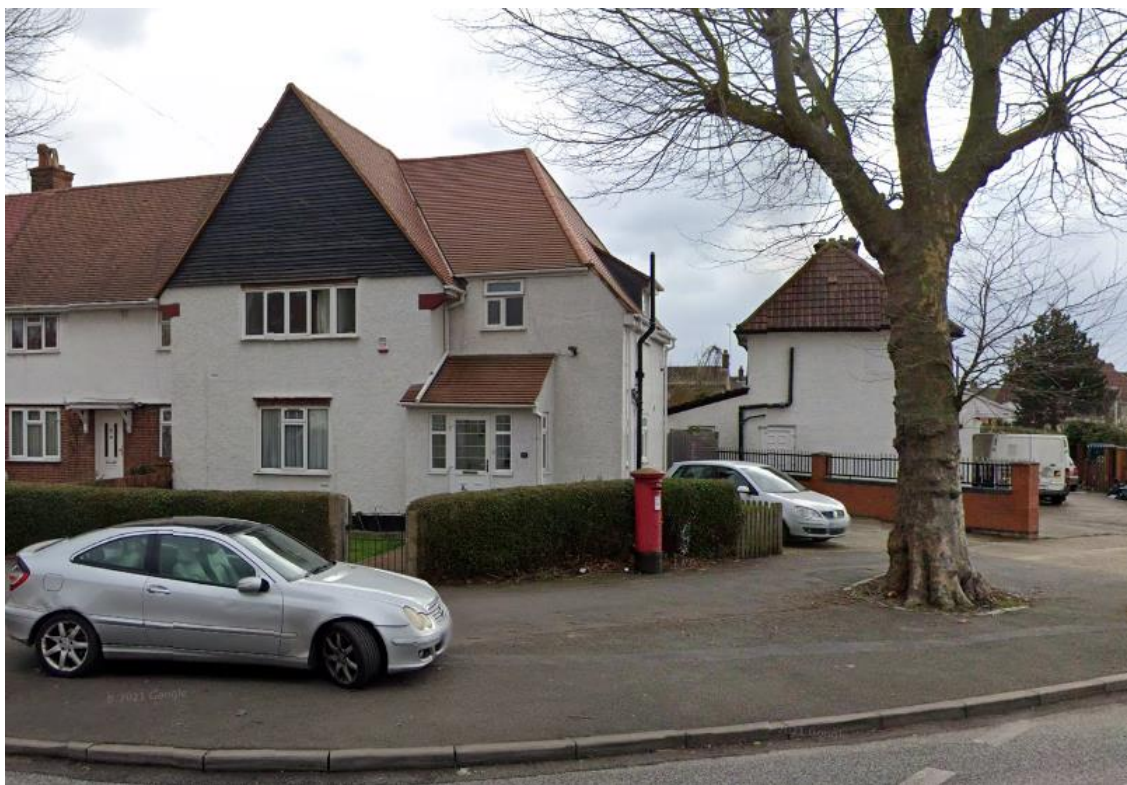
Existing extensions at no. 64 Central Avenue
