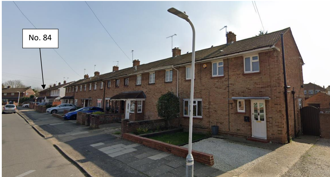
Google Street View showing host and neighbouring terrace groups
